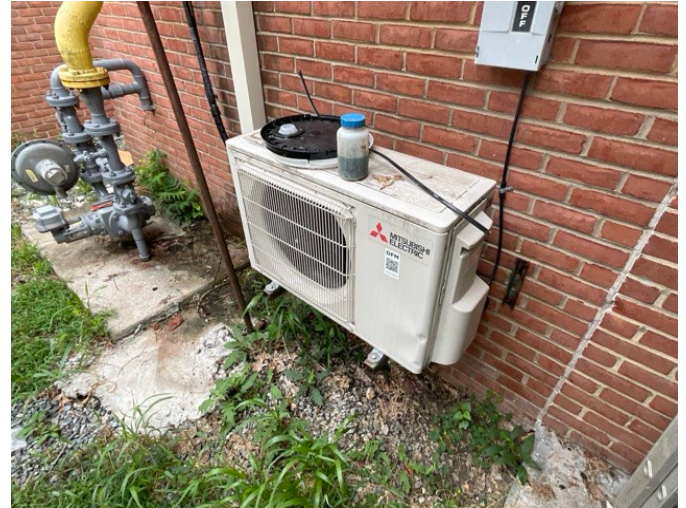
14 - SPLIT SYSTEM DUCTLESS
