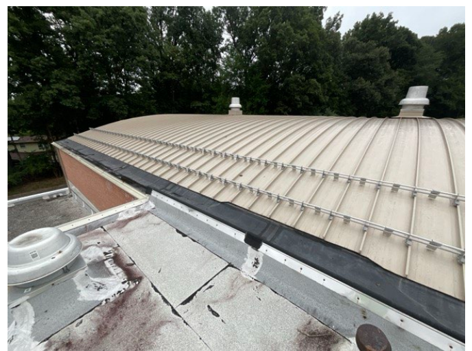
6 – MODIFIED AND METAL ROOFING
