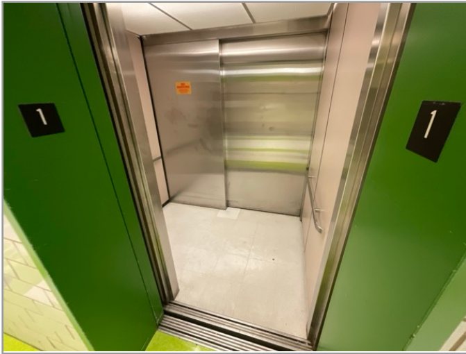
LOBBY LOOKING AT CABS
