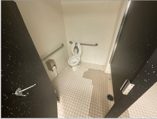
TOILET STALL OVERVIEW
