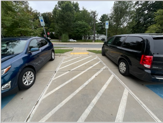
OVERVIEW OF ACCESSIBLE PARKING AREA
